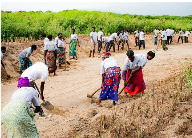
Community members from Mnembe constructing water holding trenches within their community to offset the impact of floods.
